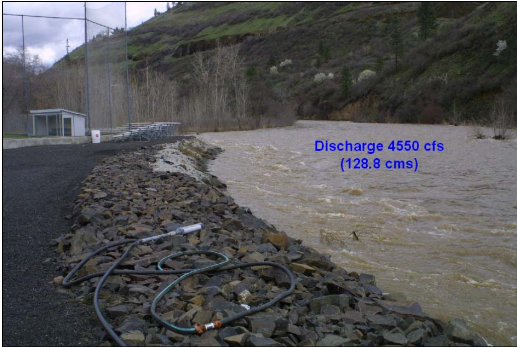
Figure 3.67 Centennial Reach at a discharge of 4550 cfs on March 31, 2005.
