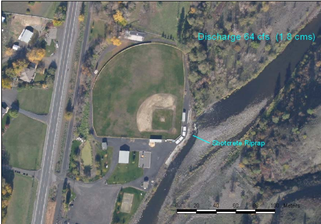
Figure 3.59 Channel bank reinforcement at the softball field (aerial).
