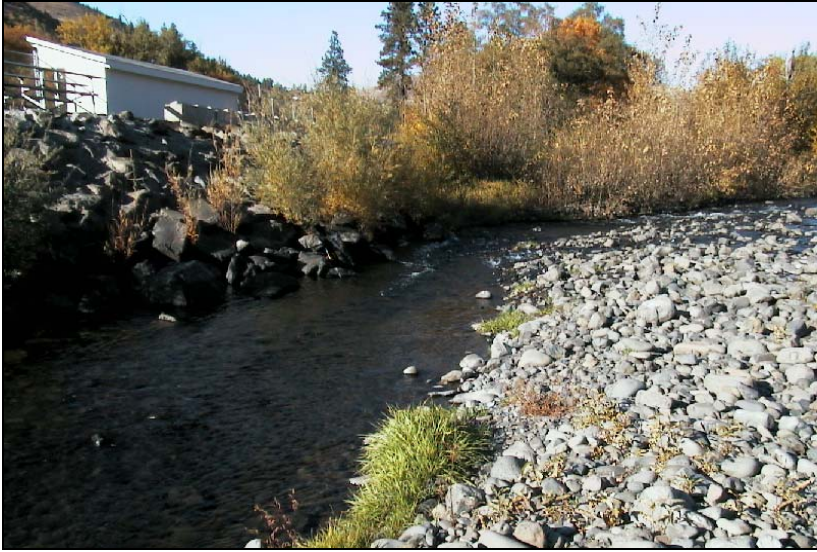
Figure 3.60 Channel bank reinforcement at the softball field (ground).
