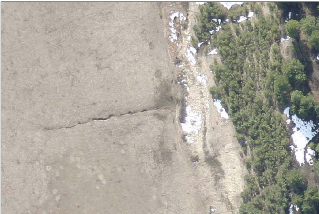
Figure 8.48 Classical gully extending upslope by seepage erosion
