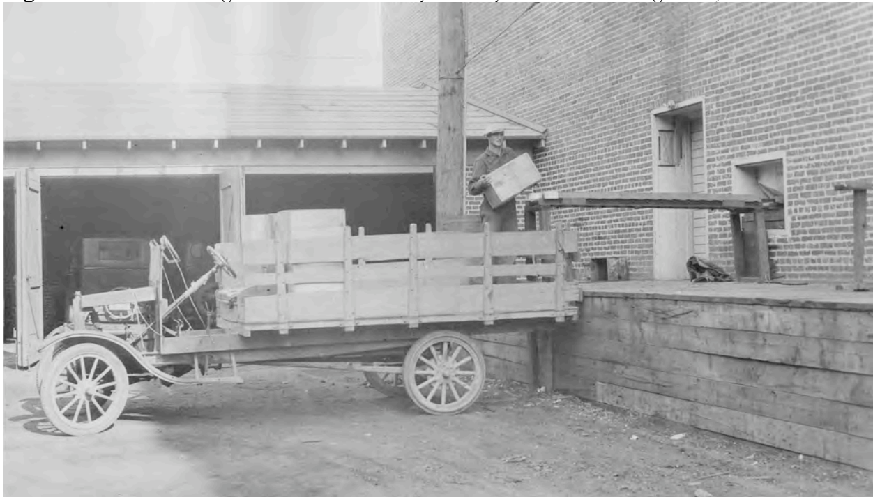
Figure 6.13. Unloading a Truck onto Gravity Conveyors at the Packinghouse, c. 1925.
