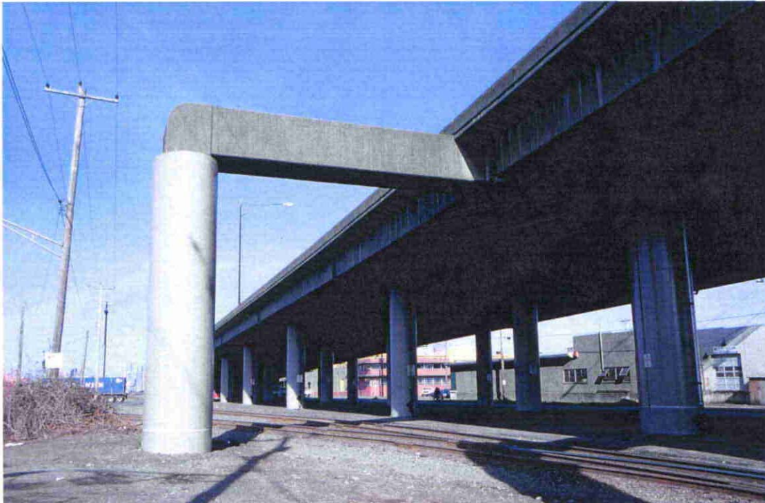
Figure 1.1 Outrigger Bent in the SR 99 Spokane Street Overcrossing
