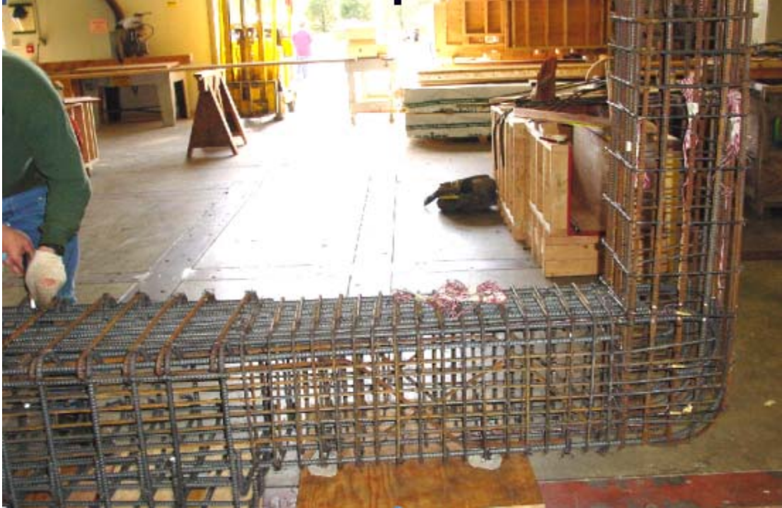
Figure 3.9 As-Built Long Outrigger Specimen Prior to Forming
