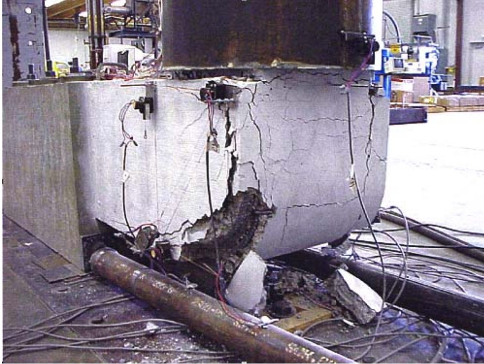
Figure 4.15 Concrete Spalling off as a Result of Splitting Bond Failure of the Column Reinforcement Within the Joint of Specimen ASI
