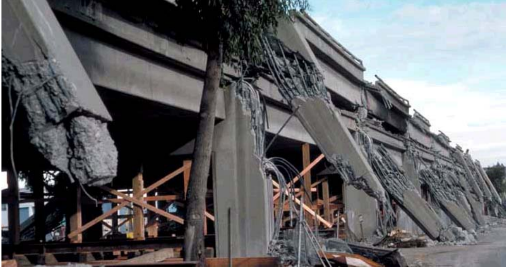
Figure 2.1 Cypress Viaduct After Loma Prieta Earthquake http://www.sfmuseum.org/1989/89photos.html
