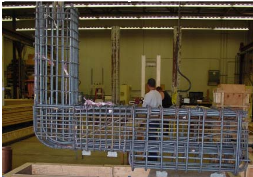
Figure 3.13 As-Built Short Outrigger Specimen Prior to Forming
