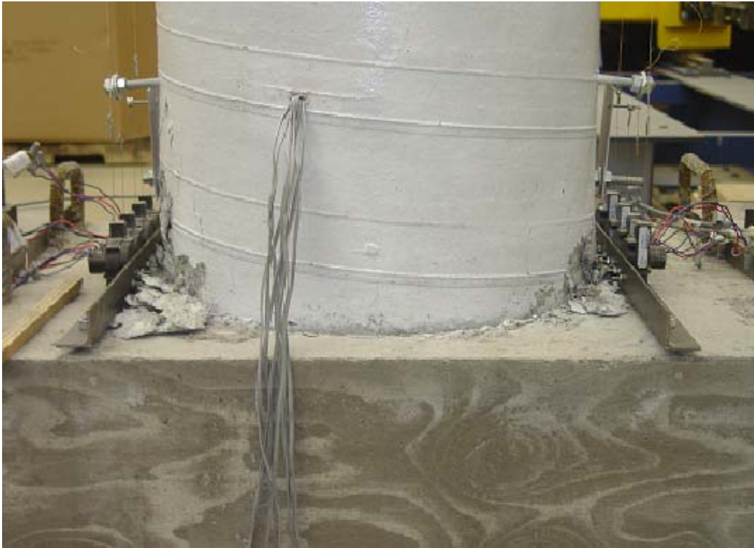
Figure 3.4-6 Final State of Damage for Column
