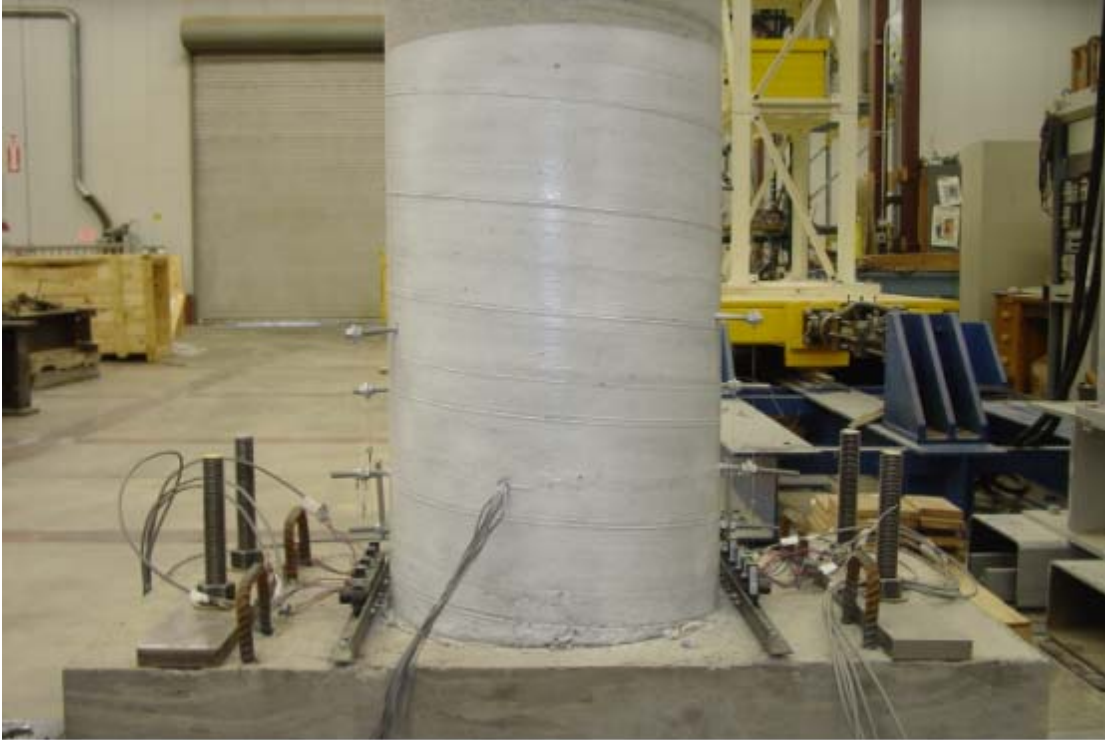
Figure 5.2-16 Final State of Damage in Column
