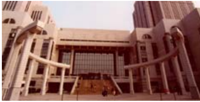
Figure.84. Main entrance with a reinterpreted of western colonnade.
