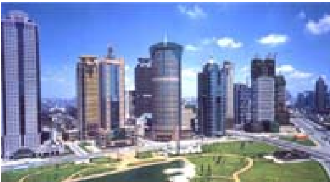
Figure.64. Commercial buildings with various styles dominate the urban landscape of Shanghai.
