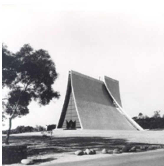
Figure.47. Luce Memorial Chapel. The profile of the concrete curve wall signifies a traditional pagoda roof.
