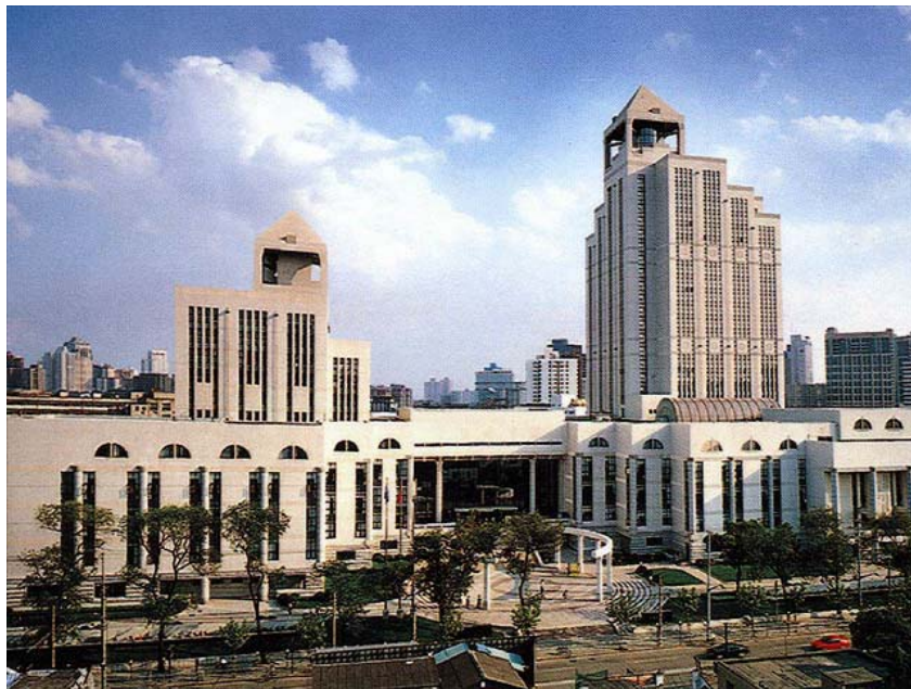
Figure.78. The setback layout breaks the mass volume and forms a rich roofline.
