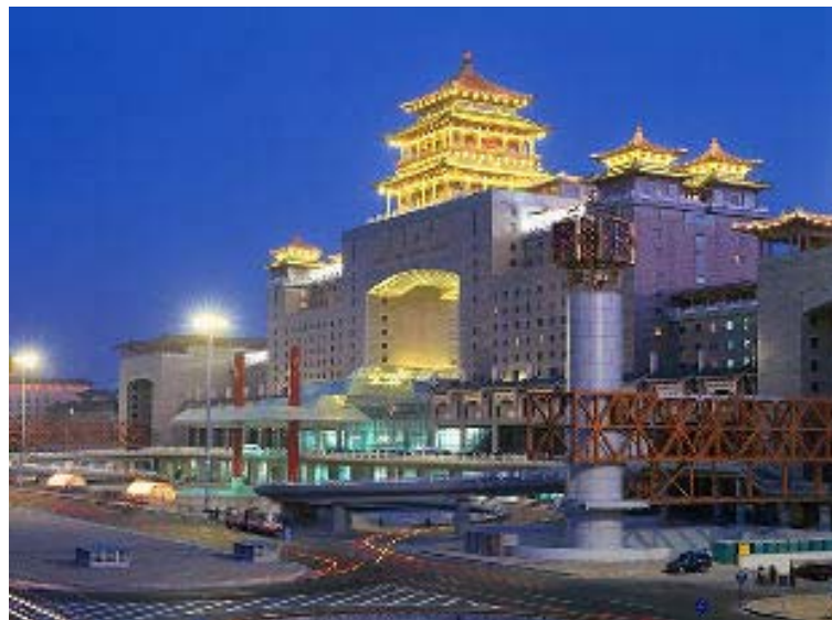
Figure.4. The Beijing West Railway Station is a typical example of misuse of traditional forms.
