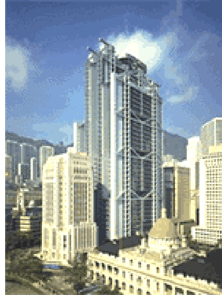
Figure.98. Details of Hong Kong Bank demonstrates technological aesthetics.
