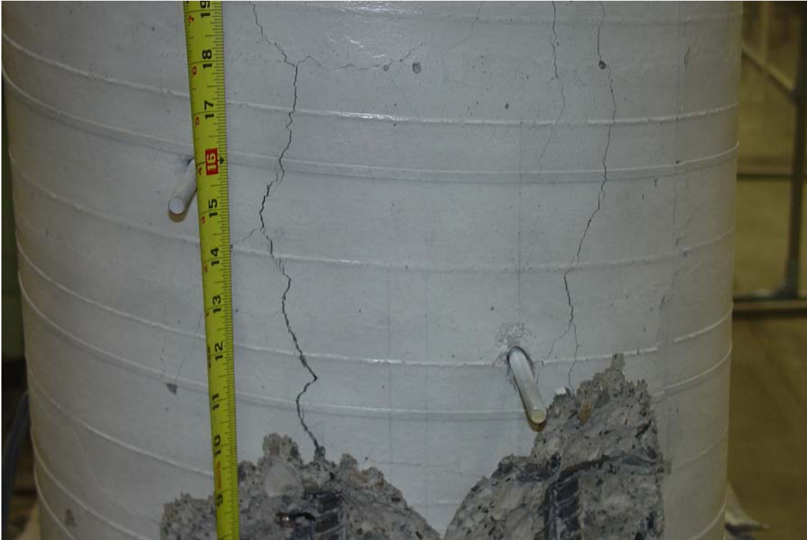
Figure 6.1-12 Vertical Cracks at Tension Face (Stapelton, 2004)
