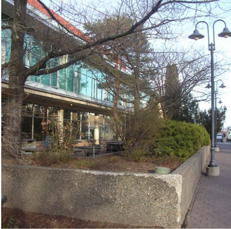
Figure 11. Planter surrounding the Compton Union Building patio
