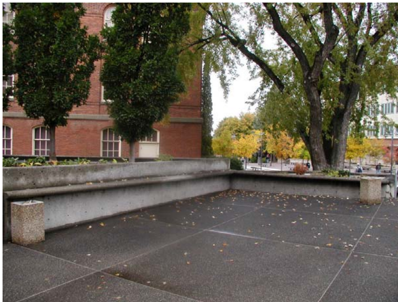
Figure 7. Concrete bench on Todd Hall's front porch
