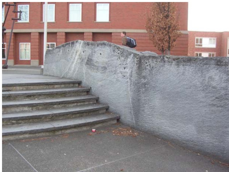
Figure 9. Quarried stone positioned on its side
