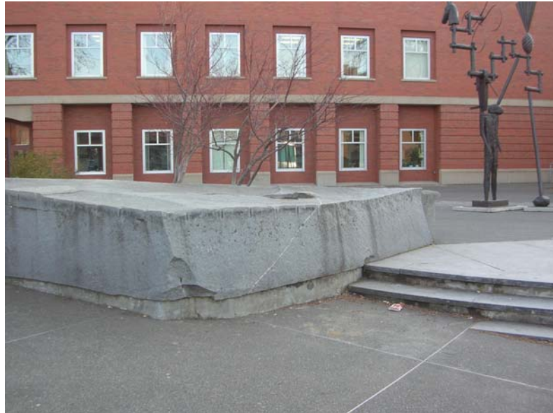
Figure 8. Large quarried stone and curved steps on Todd Hall's front porch
