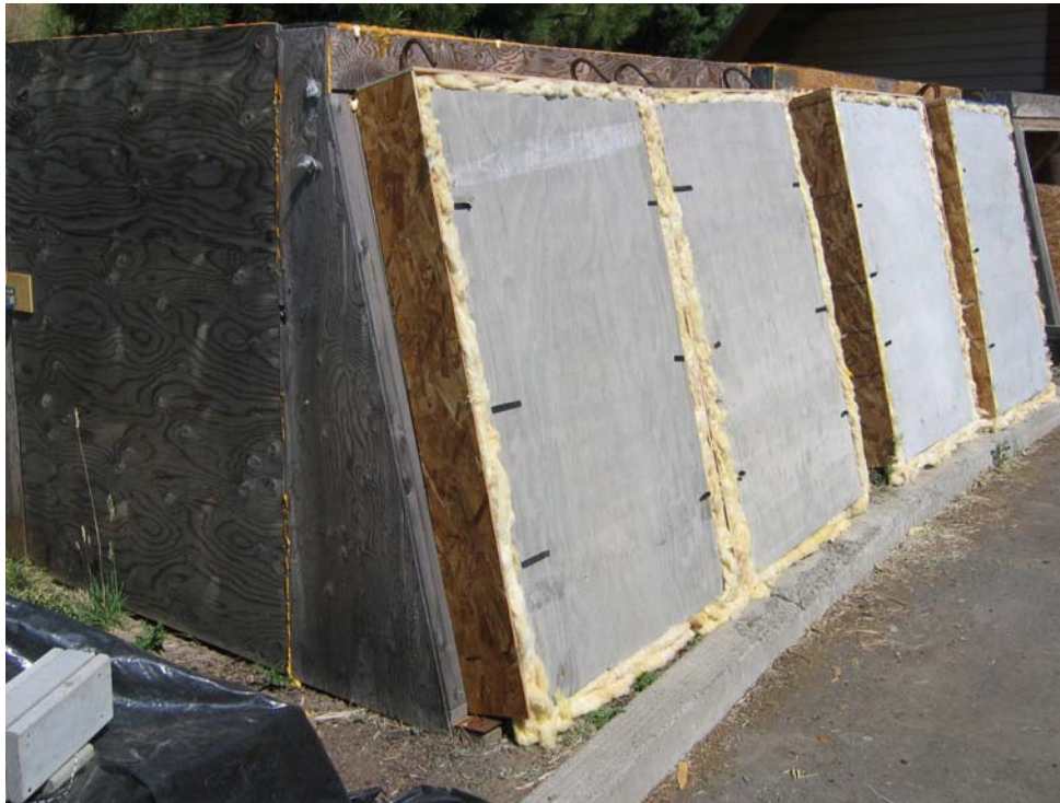
Figure 4.4 – Insulating barriers installed on the specimens
