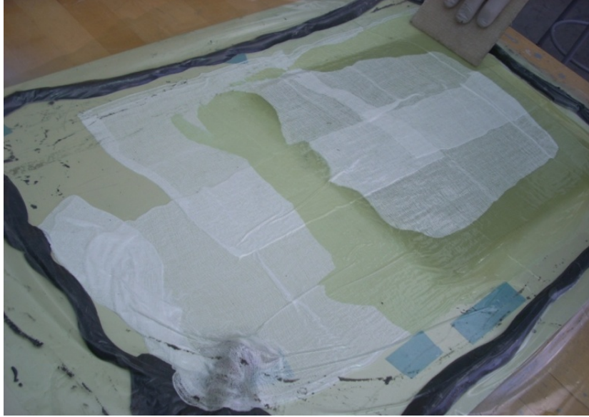
Fig 4.2-14: Vacuum Taking Effect on Prepared Lay-Up
