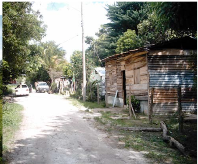
Figure 4. A typical plywood and nail house with a tin roof.
