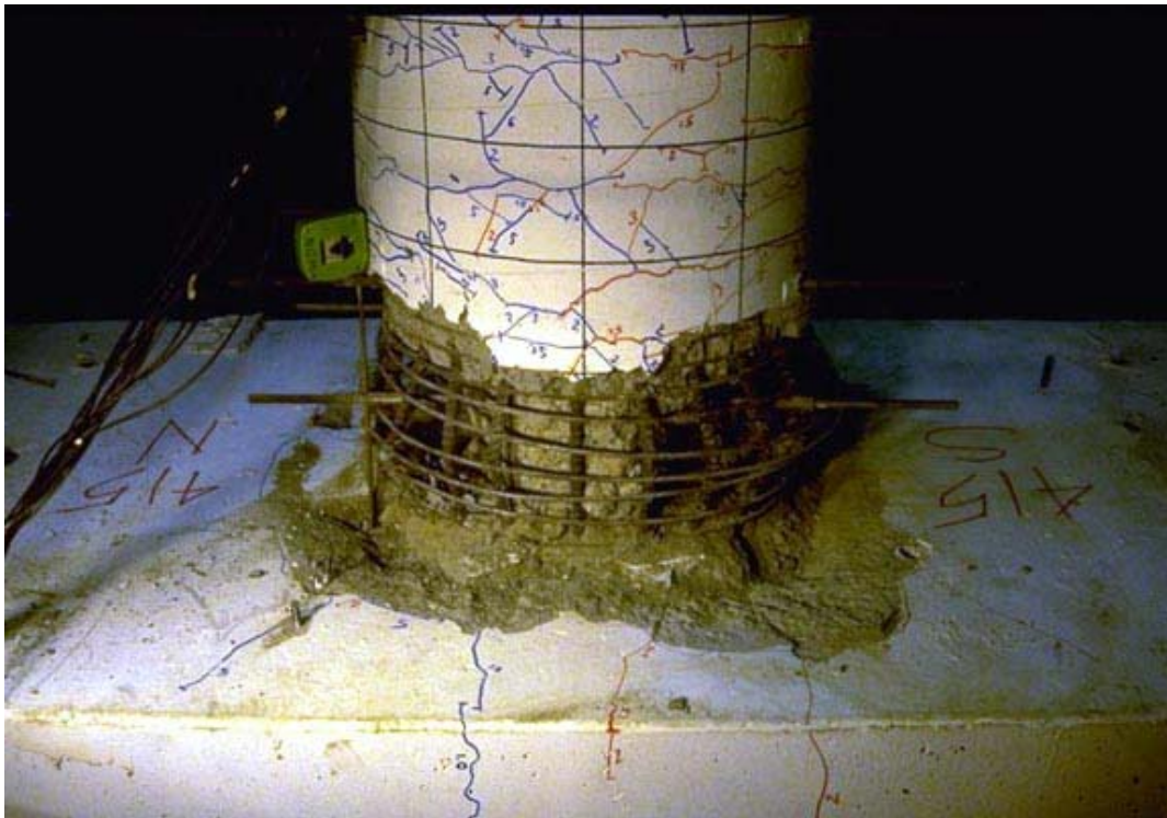
Figure 3.2.4: Final damage state (Lehman, 2000)
