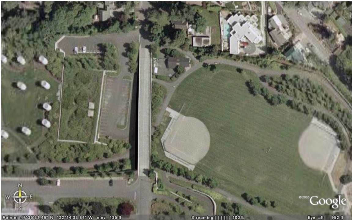
Figure 4.6.2: Bridge 90 Aerial Views
