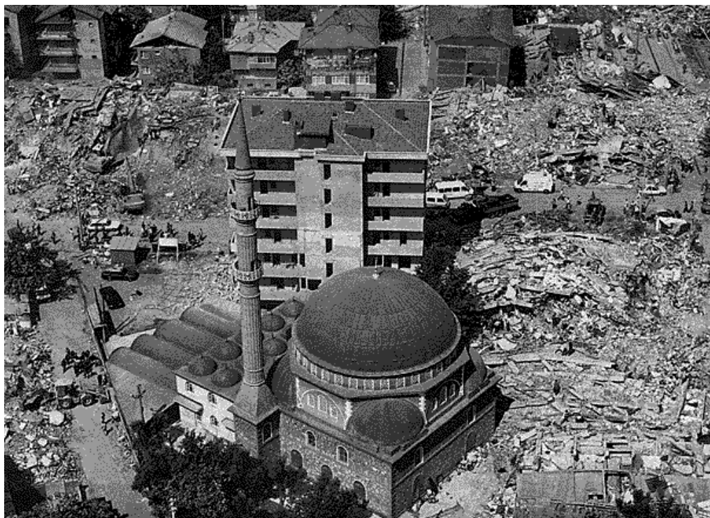
Figure 5.1.11: A mosque stood with a few other structures amid the rubble of collapsed buildings in the town of Golcuk, 60 miles east of Istanbul (Associated Press Photo, Enric Marti, 1999).
