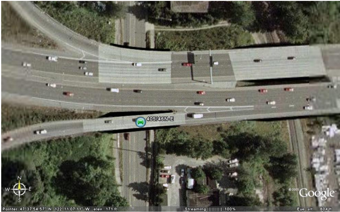
Figure 4.4.1: Bridge 405 Aerial View
