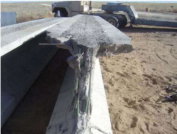
Figure 4-5: Web Cracking-Blast Above, Experimental
