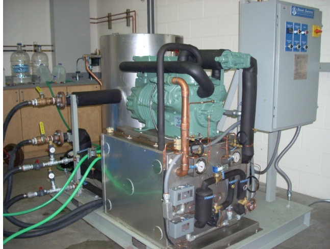
Figure 3.5 Packaged water-cooled chiller.
