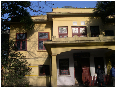
Fig.17. Main Façade of Chenlu (by Qi,Q.,2005)
